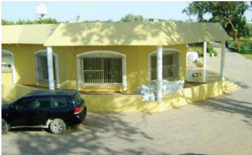
A sandbag fighting position on the Compound, before September 11, 2012. (State Department photo)
