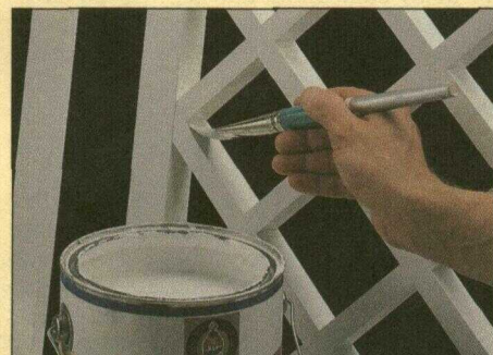
Exterior Latex Paint. After the latticework is nailed in place, I touched up the holes with spackling and exterior latex paint.
